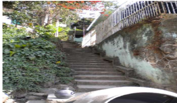
Calle Aconcagua: possible drainage project
